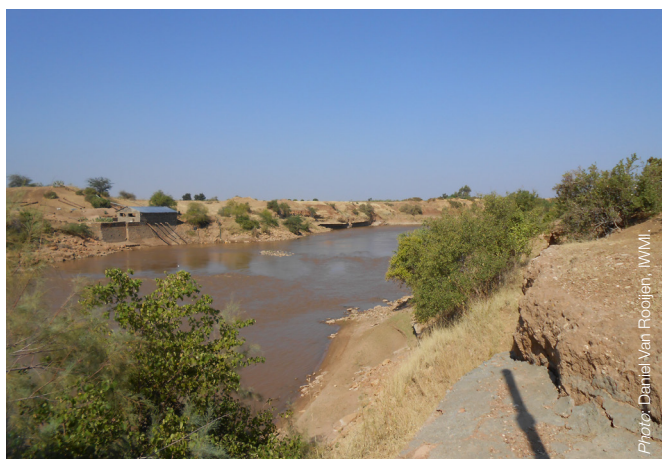
View of the Shebelle River and water intake station in the arid lowlands.
