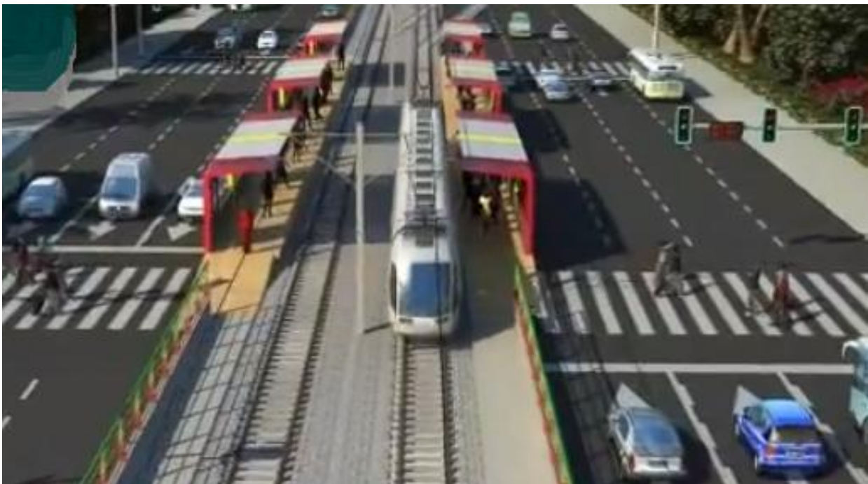
3D Simulation of the Addis Ababa Light-Rail Transit System - which involves the construction of the 34.25 km double track electrified light rail transit. The transit system which is to be completed in 2015 will provide transportation service to 60,000 people per hour.
